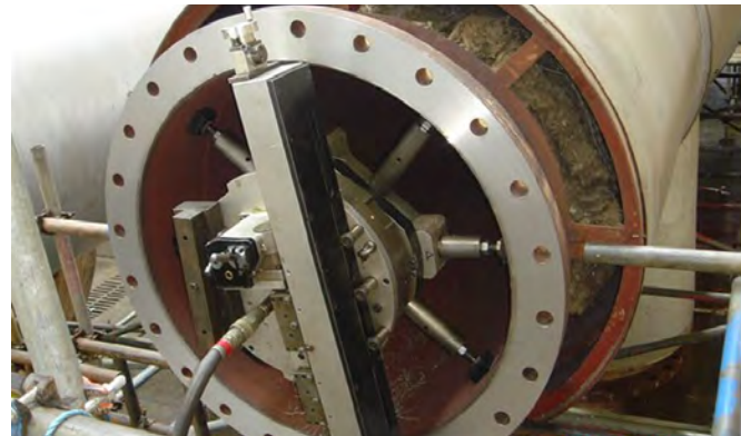
2M Ø Flange being machined perfectly flat
