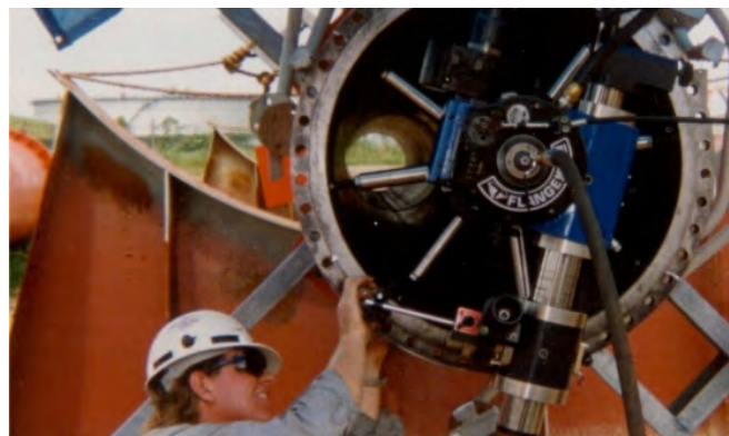
Setting Up The Flange Facer to Machine A 650mm Ø Flange
