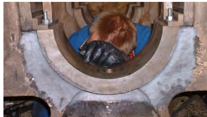
Finished Repair After Hand Dressing
