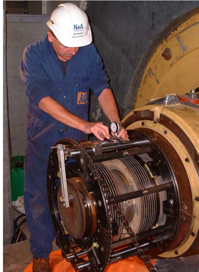
Machining Sliprings in a Power Station
